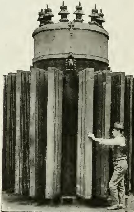
The Largest Self-control Induction, Feeder Voltage Regulator Ever Built.
