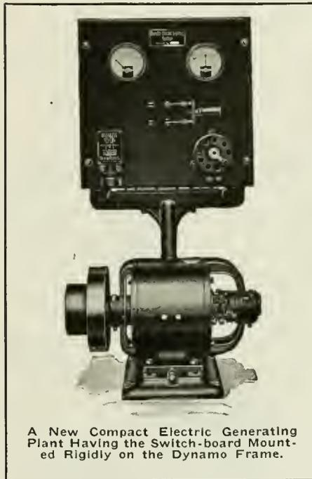
A New Compact Electric Generating Plant Having the Switch-board Mounted Rigidly on the Dynamo Frame.
